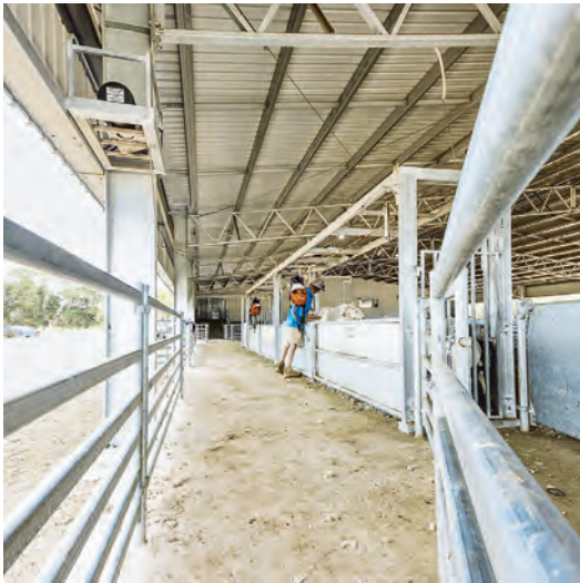
A roof over yards provides good working conditions year-round and flexible working hours, increasing productivity and labour efficiency.
